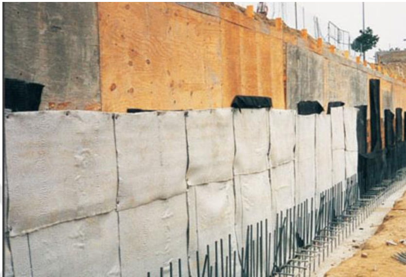
Hydro Clay (applied as membrane and hydrated)
